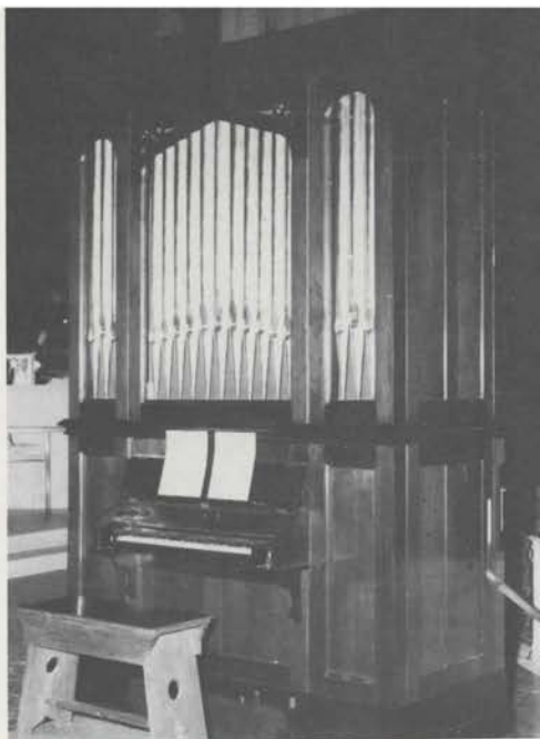
This tracker action organ at Grace Cathedral was built about 1860.
