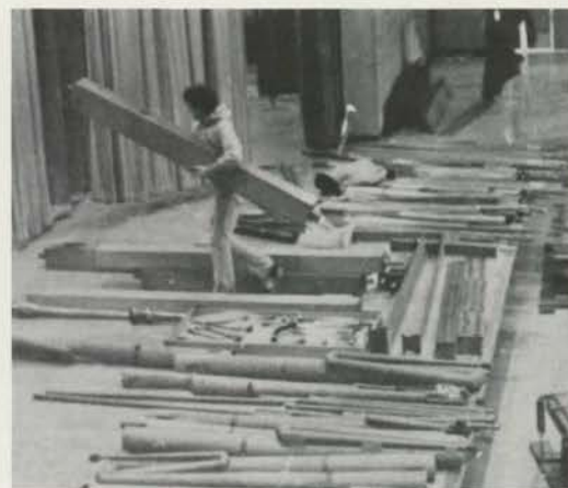
Pipes laid out on stage.
