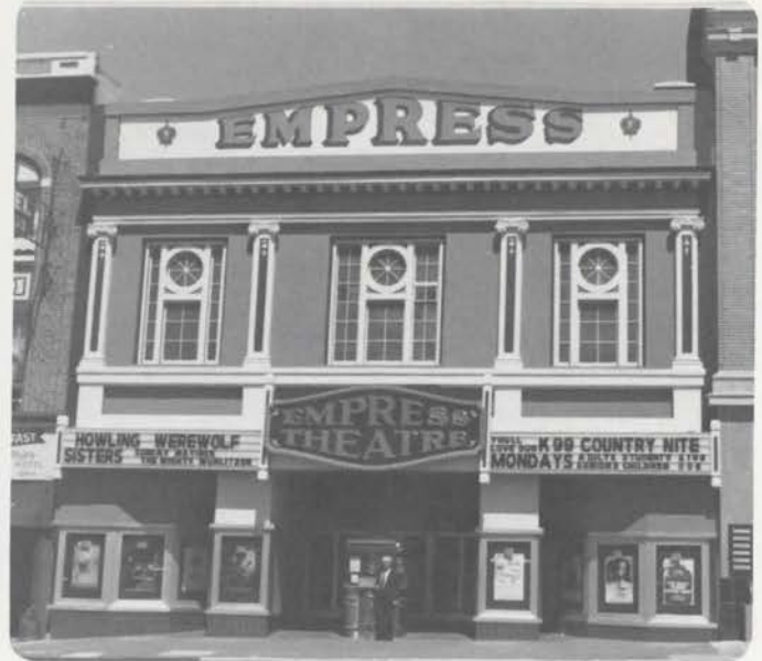
Facade of the Empress Theatre, Vallejo, California.
