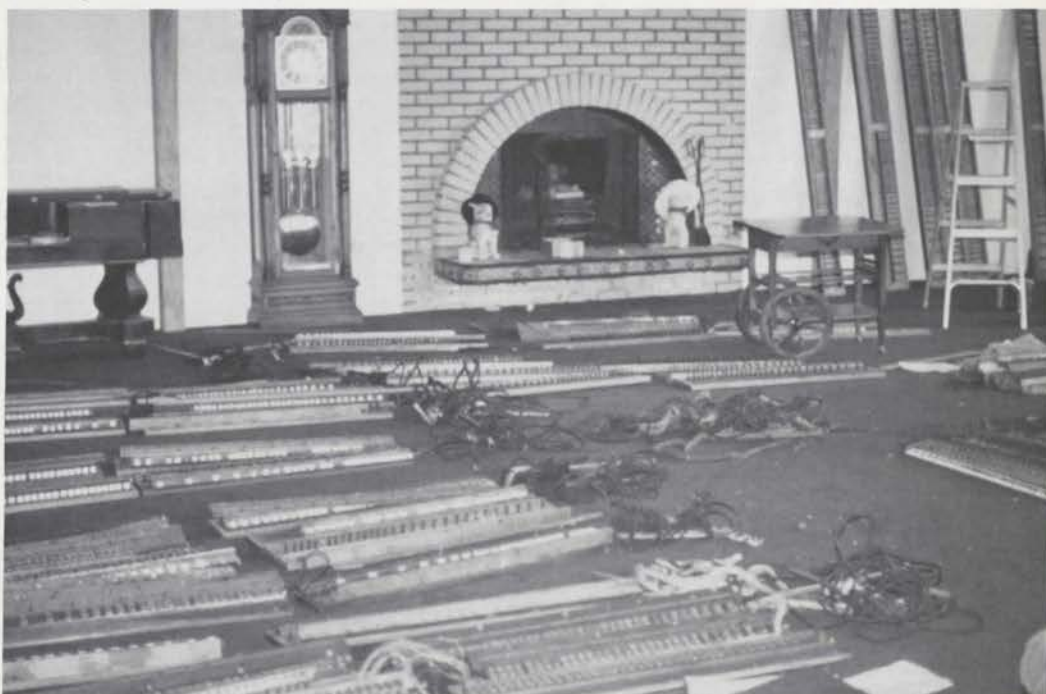
Living room during early stages of rebuilding.
