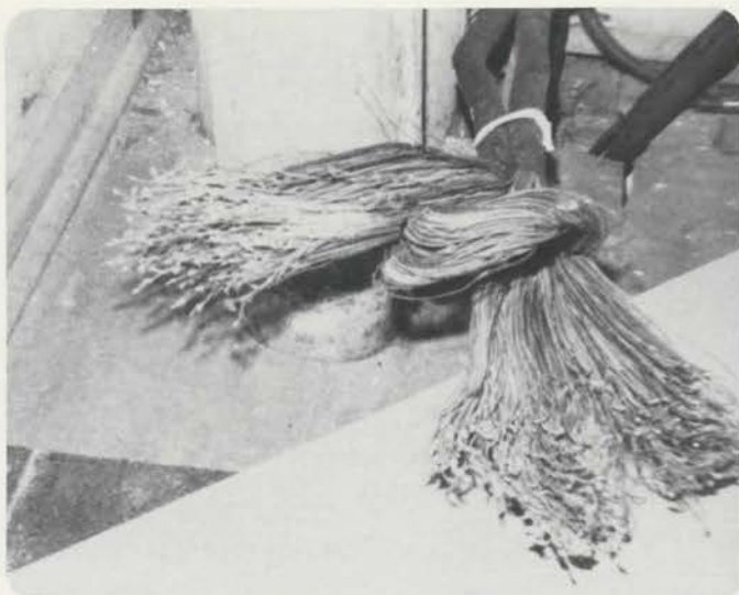
Cut cable at the Denver Aladdin Theatre, 1983.
