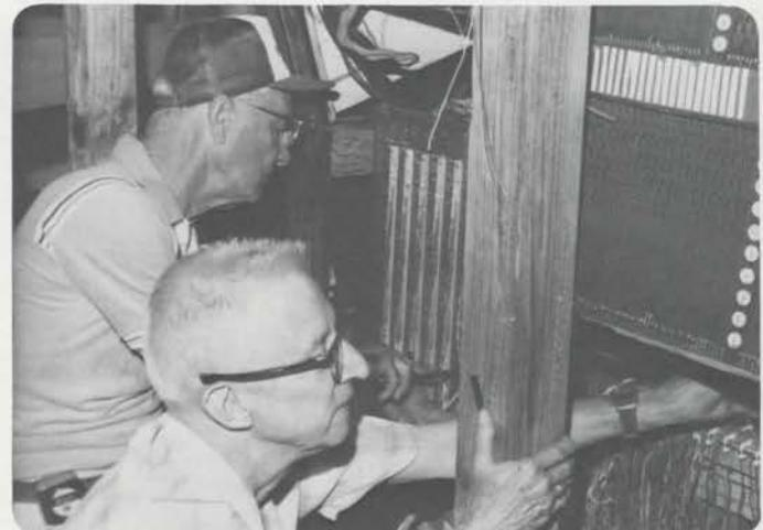
Lee Wilson, rear, and Ed Lawrence checking the wiring and solid-state units in the console of the 3/12 Wurlitzer which CFTOS is installing in the Tampa Theatre. (John Otterson photo)
